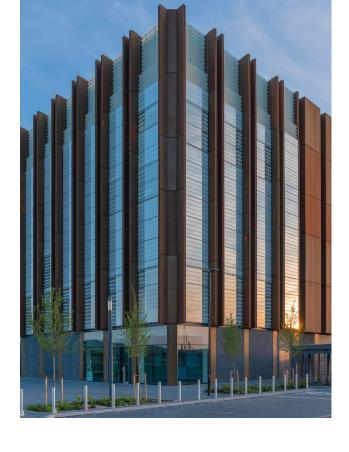
manufacturing and fabrication machinery to produce 7,800m<sup>2</sup> of COR-TEN steel and then specialist jigs and trollies were used to assemble the oversized modular units and safely and efficiency transport them around the factory and onsite.
